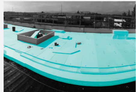
Achieving proper roof slope with FIBRANxps INCLINE and installation of FIBRANxps boards on a non-ballasted roof.
