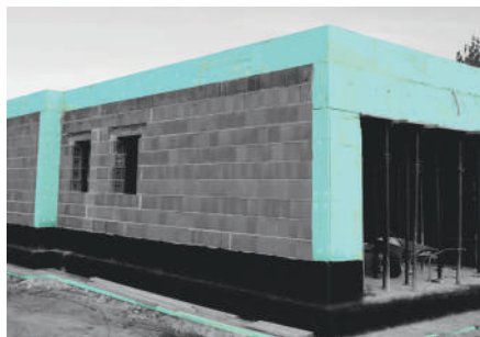
Insulation of thermal bridges on tie beams with FIBRANxps ETICS .
