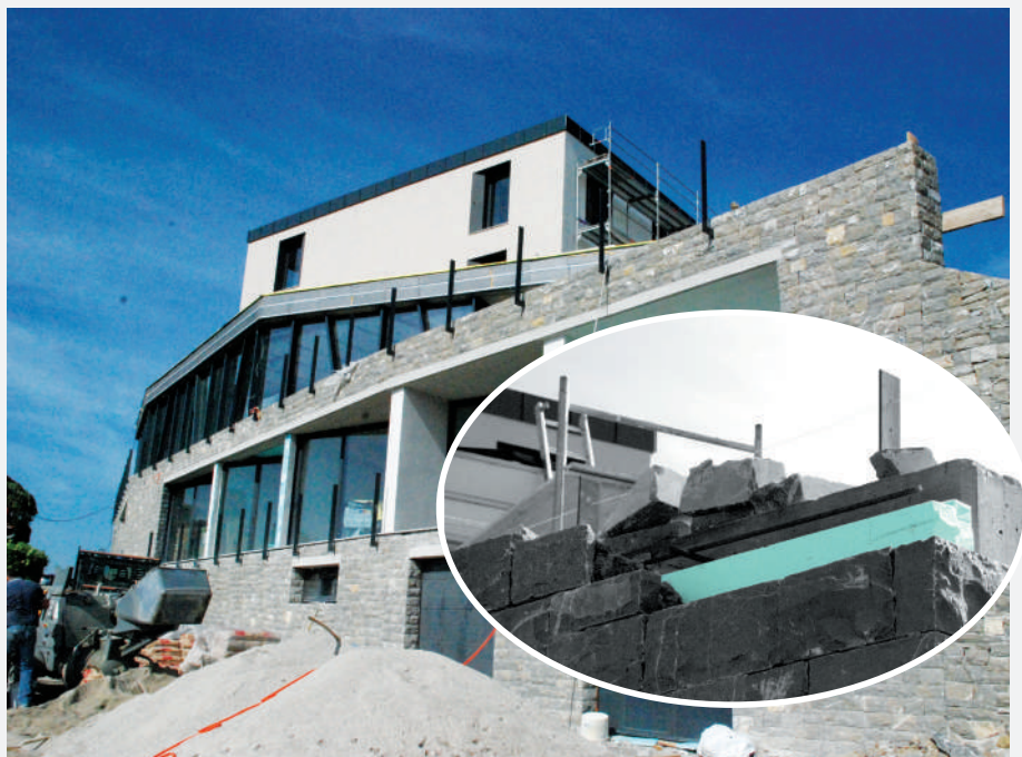
Stone cladding of a hotel building insulated with load-bearing insulation FIBRANxps ETICS BT , to which natural stone is attached with adhesive using a special procedure.
