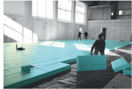
Fitting of thermal insulation FIBRANxps 500-L underneath foundation slab of multi-functional building.
