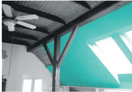
Interior thermal insulation rendered with FIBRANxps ETICS , surface protected with coatings of thin-layered render and paintwork.
