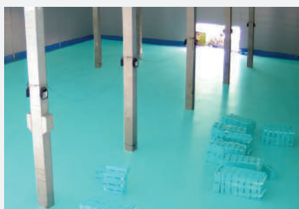
Thermal insulation of a cooling warehouse with FIBRANxps 500-L , 700-L .
