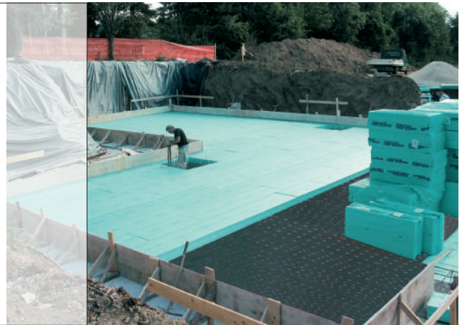
Detail 7 - Because of the »load dispersion rule is chosen, as shown in the detail. Preparation of thermal insulation base of a residential building.
