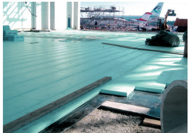
Thermal protection of the ground of airplane hangar with FIBRANxps 700-L.
