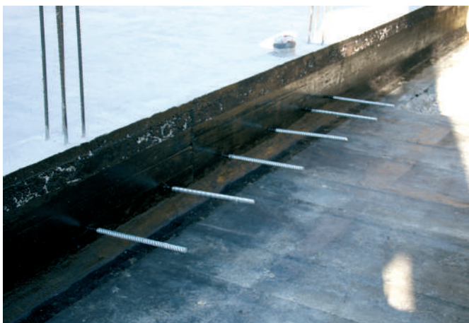
Detail 3 - Prefabricated elements, such as light shafts are installed according to the manufacturer's instructions. The penetration, caused by anchoring the light shaft, needs to be carefully sealed. The part of the construction should be thermally insulated from cold construction of light shaft.
