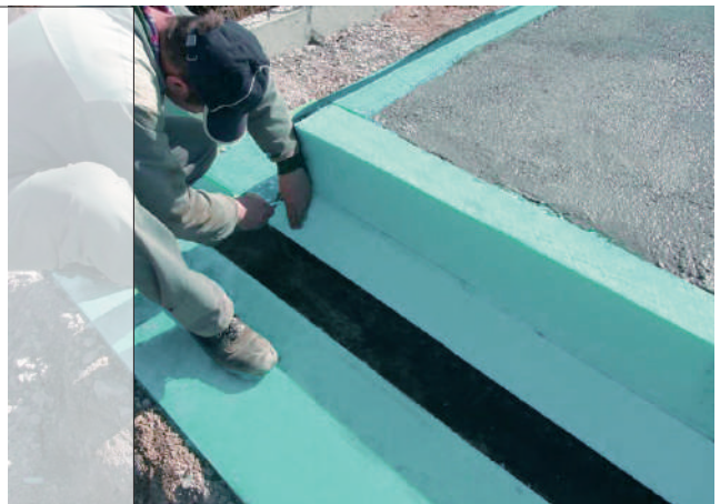
Detail 9 - Waterproofing between two layers of FIBRANxps 400-L insulation boards. Application of an angle fillet to smooth the inside corners of vertical bituminous waterproofing.
