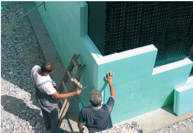
Cross instalation of FIBRANxps 300-L boards and fitting of junctures.
