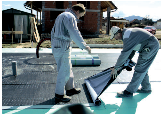
Laying of self-adhesive waterproofing on thermal insulation boards FIBRANxps 400-L.
