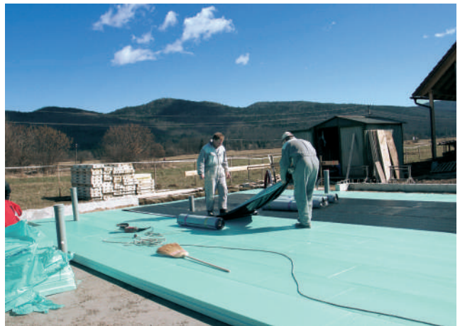
Self-adhesive waterproofing between two layers of FIBRANxps 400-L thermal insulation.
