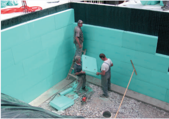
Gluing of FIBRANxps 300-L boards with butyl rubber stickers FIBRANstick.
