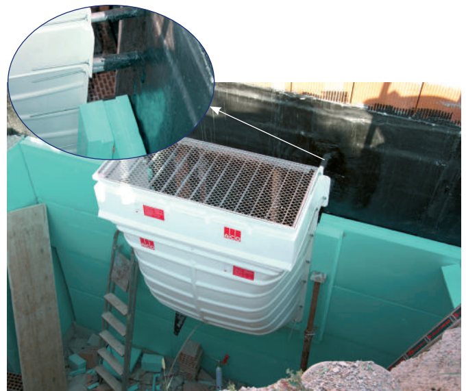
Detail 3 - Prefabricated elements, such as light shafts are installed according to the manufacturer's instructions. The penetration, caused by anchoring the light shaft, needs to be carefully sealed. The part of the construction should be thermally insulated from cold construction of light shaft.
