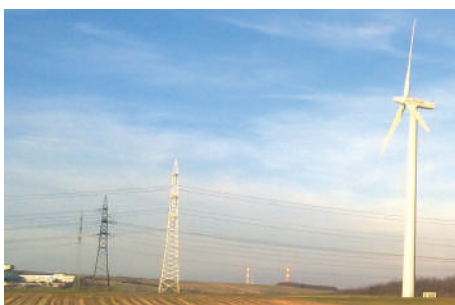
Thermally insulated ground around foundations ensures stability of constructions exposed to temperature fluctuations.
