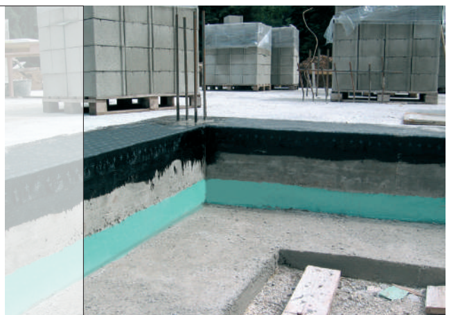
Detail 10 - Bituminous waterproofing on the foundation slab of a building with basement. Thermal insulation FIBRANxps 400-L underneath the foundation slab.
