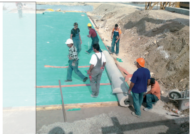
Detail 8 - Ecological bentonite waterproofing placed on FIBRANxps 400-L before building the foundation slab of a school building.
